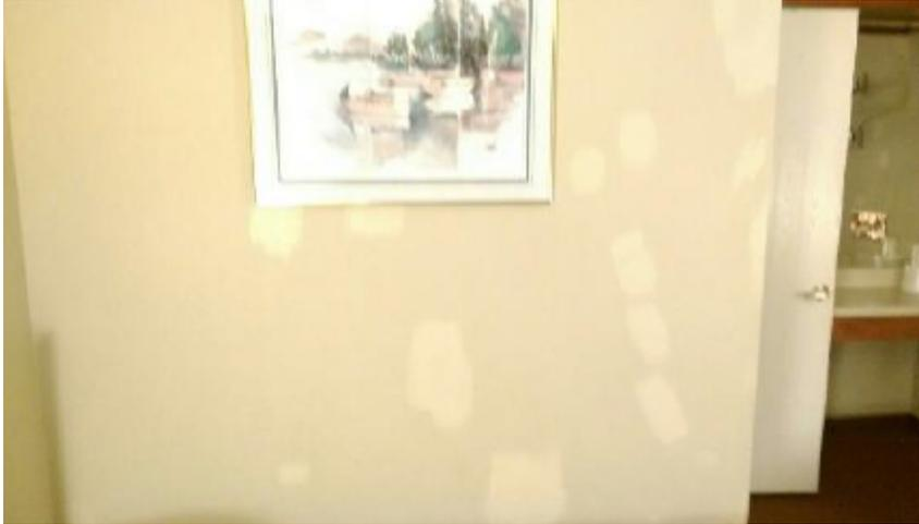
3. **Touch-up was done instead of painting full walls:** If painting is necessary, touch-up painting can be problematic, and in many cases painting entire select walls may be necessary. This applies if the paint color and sheen are not close enough of a match.
